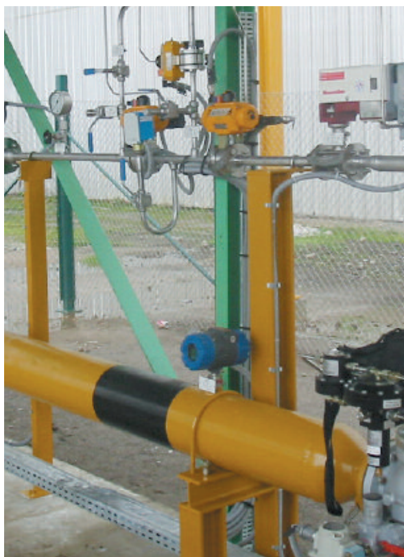
Bio-gas, a mixture of methane and carbon dioxide, results from the decomposition of organic materials and can be harvested as a fuel source. Due to its low flow sensitivity and low pressure drop, the TA2 is an excellent flow meter for measuring bio-gases.
